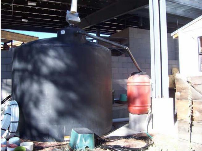
This rainwater collection tank is used for watering the garden. This water comes off the roof of the CCC kiln.
